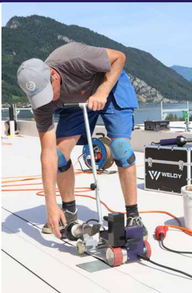
123.287 Overlap welding nozzle, 40 mm
